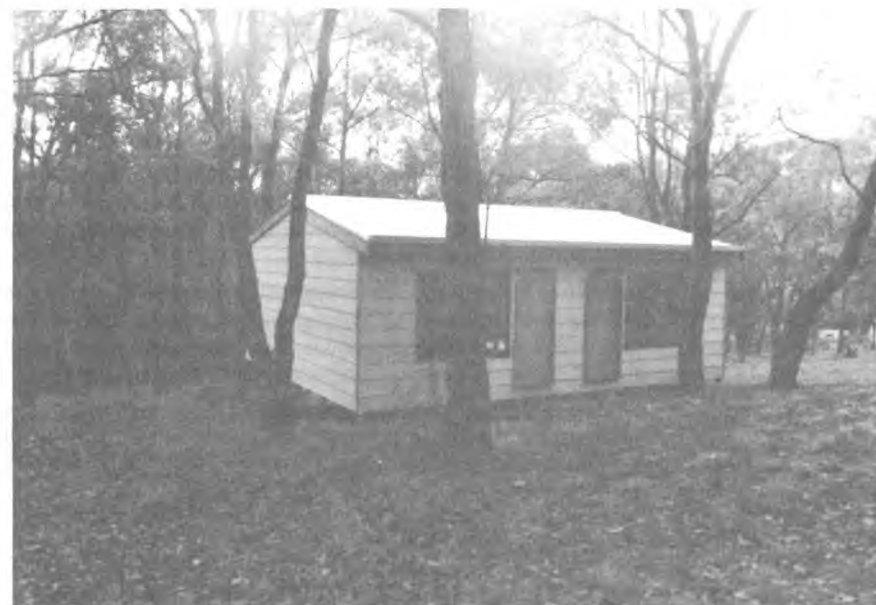
Woori Yallock Accommodation Unit, 1980.
