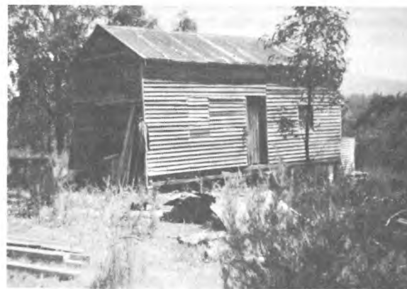
Woori Yallock: The first building, 1950; still in use as the kitchen, 1980.
